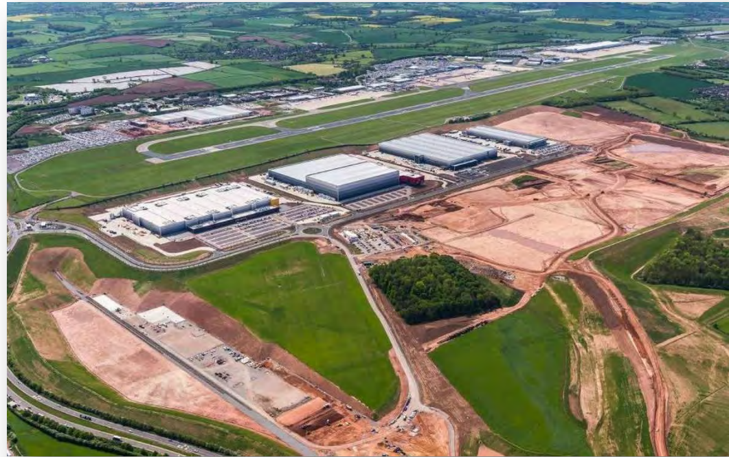
Figure 5: SEGRO Logistics Park East Midlands Gateway under construction (image: PHP Architects)
