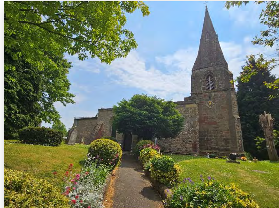
Figure 15: St Michael's Church, Diseworth- Grade II* Listed
